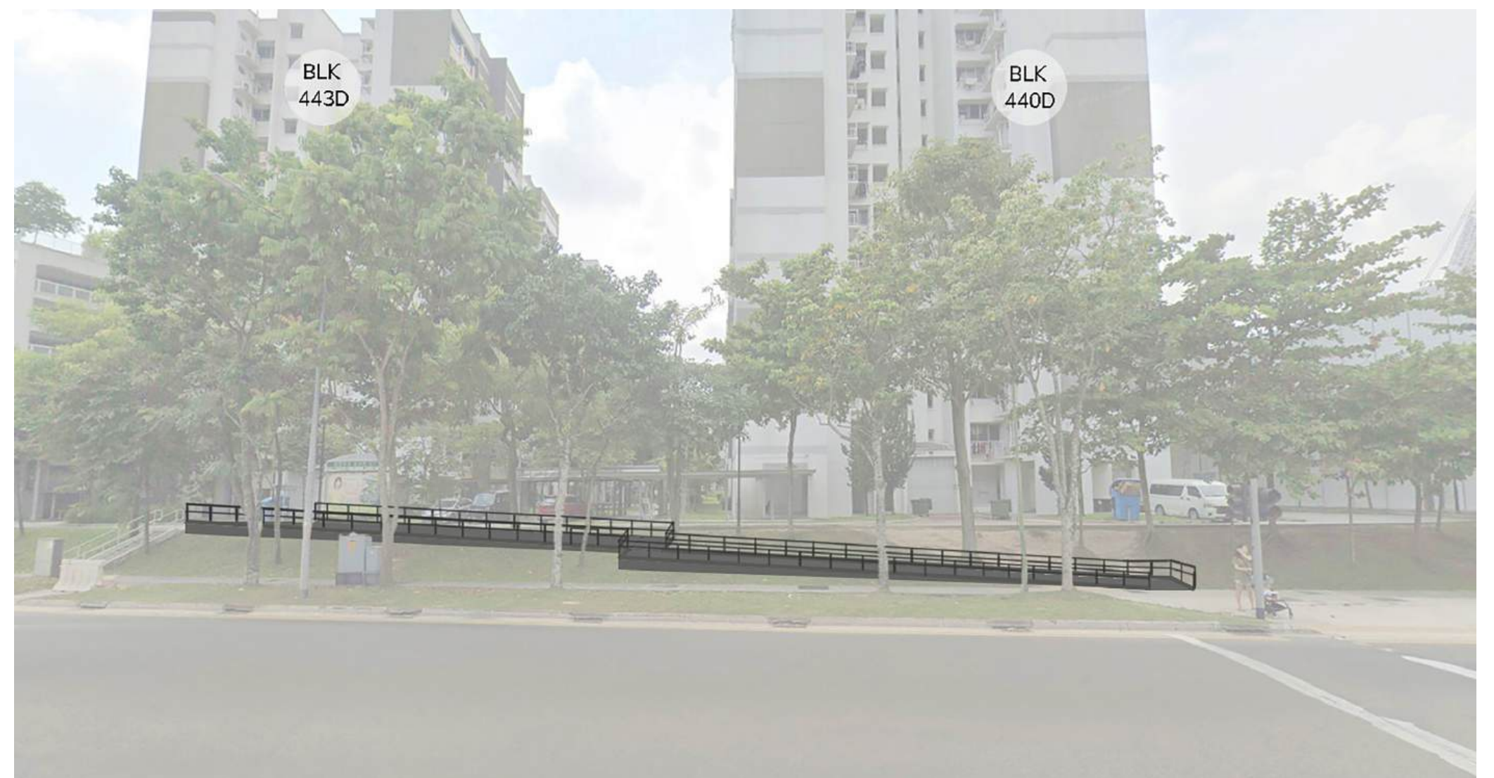
New Barrier-free Access Ramp at Block 443D Bukit Batok West Ave 8
