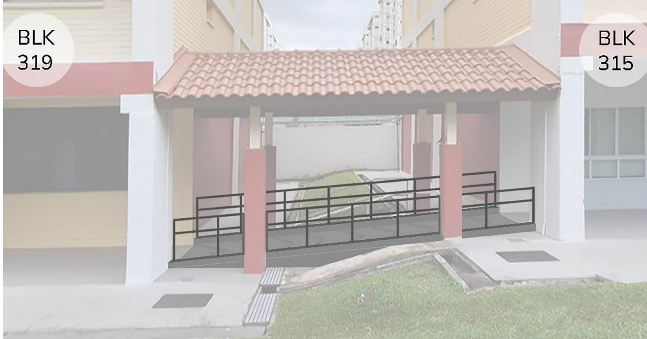
New Barrier-free Access Ramp from Block 315 to 319 Bukit Batok St 32
