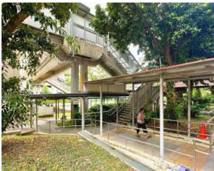
NEW COVERED LINKWAY BETWEEN BLOCK 642 BUKIT BATOK CENTRAL TO OVERHEAD BRIDGE
