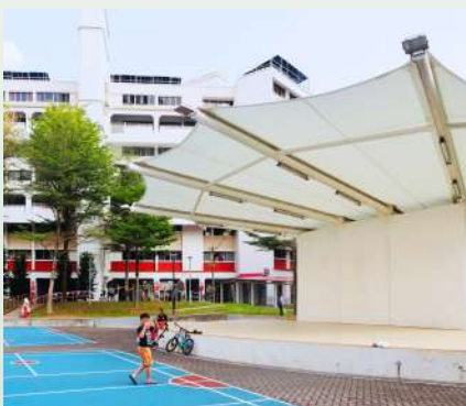
UPGRADED ROOFING FOR GALLERY, FITNESS CORNER, TOILETS AND JOGGING TRACK AT BUKIT BATOK SPORTS HUB
