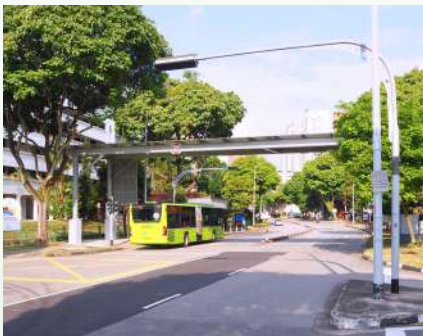
NEW HIGH LINKWAY BETWEEN BLOCK 168 AND 189 BUKIT BATOK WEST AVE 8
