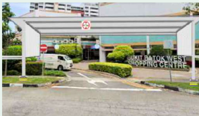
NEW HIGH COVERED LINKWAY ACROSS ST LUKE'S HOSPITAL AT BUKIT BATOK ST 11
