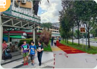
LTA'S ISLANDWIDE CYCLING NETWORK (ICN) PROGRAMME (BUKIT BATOK WEST, CLEMENTI, JURONG WEST, TAMAN JURONG)
