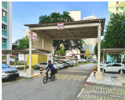
NEW HIGH LINKWAY BETWEEN BLOCK 131 AND 119 BUKIT BATOK WEST AVE 6
