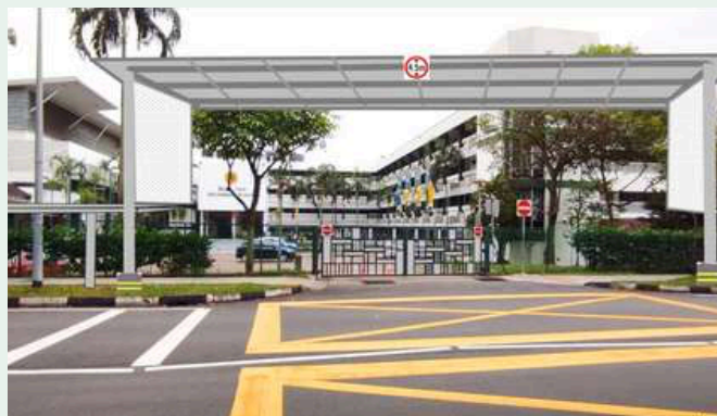
NEW HIGH COVERED LINKWAY ACROSS BUKIT VIEW SEC SCHOOL AT BUKIT BATOK ST 21
