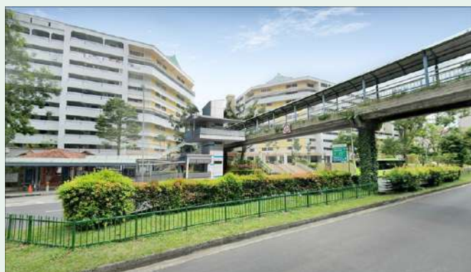
NEW LIFT AT OVERHEAD BRIDGE BLK 229 BUKIT BATOK EAST AVE 3
