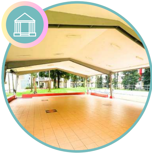
REPLACEMENT OF MPH ROOFS AT BLOCK 271, 276, 285C, 286C, 287C AND 288A
