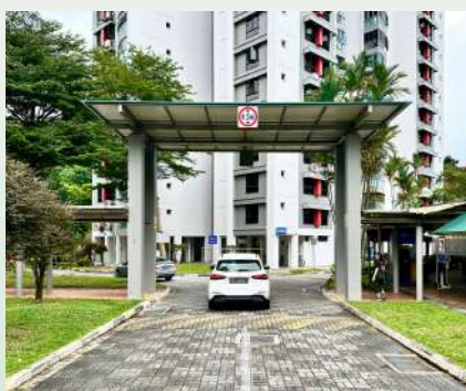
UPGRADED HIGH LINKWAY ROOF AT BLOCK 289A BUKIT BATOK STREET 25 (NATURE VIEW ESTATE)
