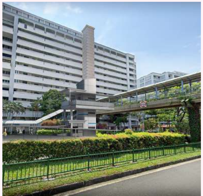
NEW LIFT AT OVERHEAD BRIDGE BLOCK 231 BUKIT BATOK EAST AVE 3
