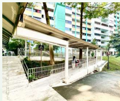
NEW COVERED LINKWAY TO EXISTING BFA RAMP LINKWAY NEAR BLOCK 254 BUKIT BATOK EAST AVE 4
