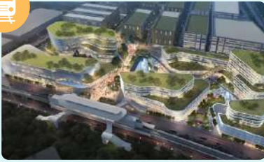
JURONG REGION LINE: NEW STATION (CORPORATION MRT STATION JS5)
