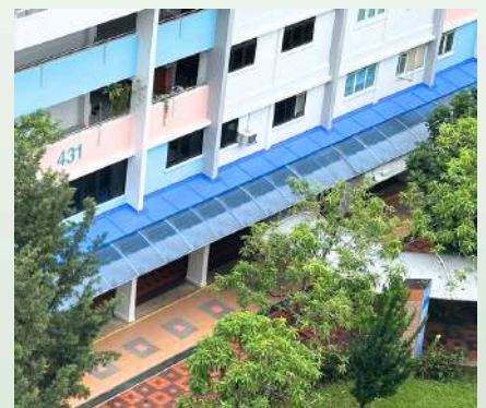
IMPROVEMENT MADE TO AWNINGS AT BLOCK 431 AND 432 CLEMENTI AVE 3
