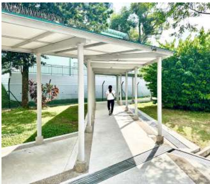
NEW COVERED LINKWAY AT BLOCK 435 CLEMENTI AVE 3 TO EXISTING LINKWAY
