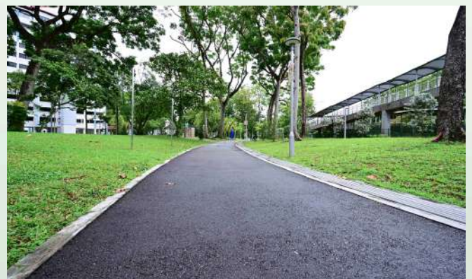
UPGRADED JOGGING TRACK FROM BLOCK 301 TO 310 JURONG EAST ST 32
