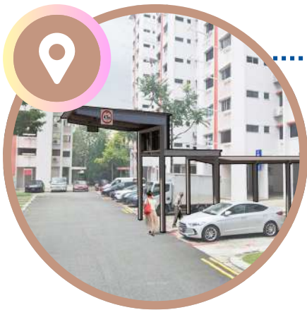
CONSTRUCTION OF DROP-OFF POINT AT BLOCK 478
