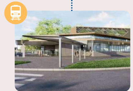
CROSS ISLAND LINE: NEW STATION (JURONG LAKE DISTRICT MRT STATION CR19)
