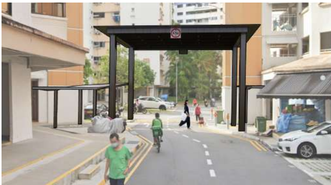
CONSTRUCTION OF HIGH COVERED LINKWAY FROM BLOCK 426 TO 428 JURONG WEST AVE 1
