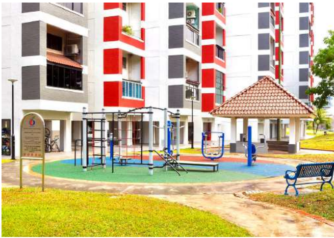
UPGRADED FITNESS CORNER AT BLOCK 407 JURONG WEST ST 42
