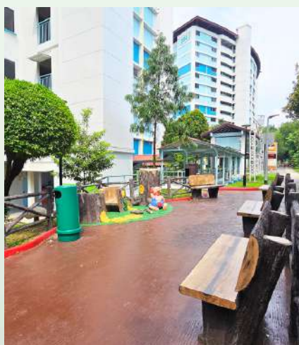
UPGRADED HARD COURT AT BLOCK 260 JURONG EAST ST 24
