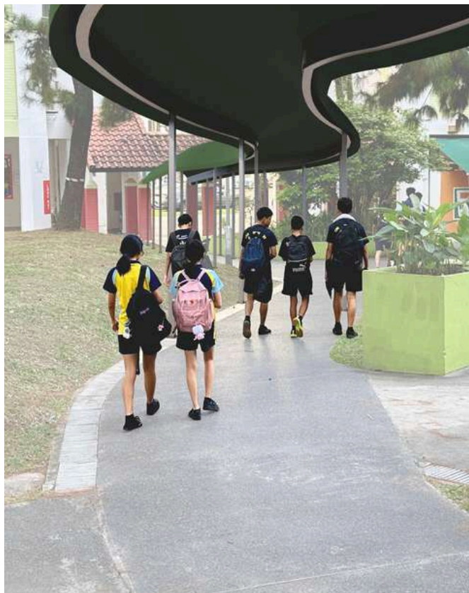
CONSTRUCTION OF LOW LINKWAY WITH RAMP BETWEEN BLOCK 243 AND 244 JURONG EAST ST 24
